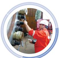
UT check before / after tensioning with tensioner
