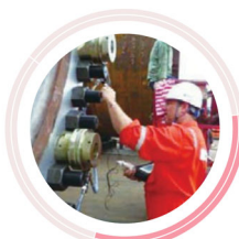
UT check before / after tensioning with tensioner
