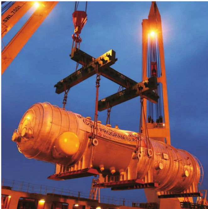
Project Shah Gas Develop.(SGD) & U.A.E Dimension 6,100ID x 30,000L, 440Ton Equipment CLAUS Package of Reaction Furnace + WHB + Steam Drum
